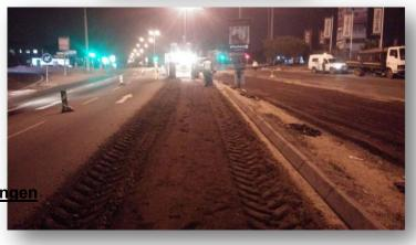
In situ stabilization/recycling of on/off-ramps, roads and driving surfaces for 2 Engen garages next to the R59. SOIL STABILISER was used due to its cost-effectiveness and speed of constructing. Minimizing traffic delays.
