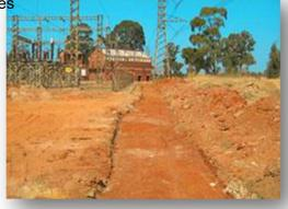
A 23km provincial road north west of Qumbu required improved selected layer support under the sub base in moist areas next to hill sides. 3.5km x 150mm thick 1% SOIL STABILISER Slab was mixed into the selected layer with considerably increased strength and water resistance. This helps to ensure adequate support for the sub base, base and bitumen seal and balances the pavement structure. This low dosage helps to prove that SOIL STABILISER can support low traffic road sub / base and bitumen seals.
